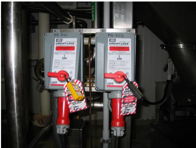
Figure 4 – The feed pump skid circuit shut off that is locked and tagged out after the incident
