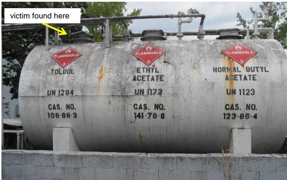
FIGURE 1: Incident site, above-ground storage tank with three 2,000-gallon sections (a. side view; b. front view).
