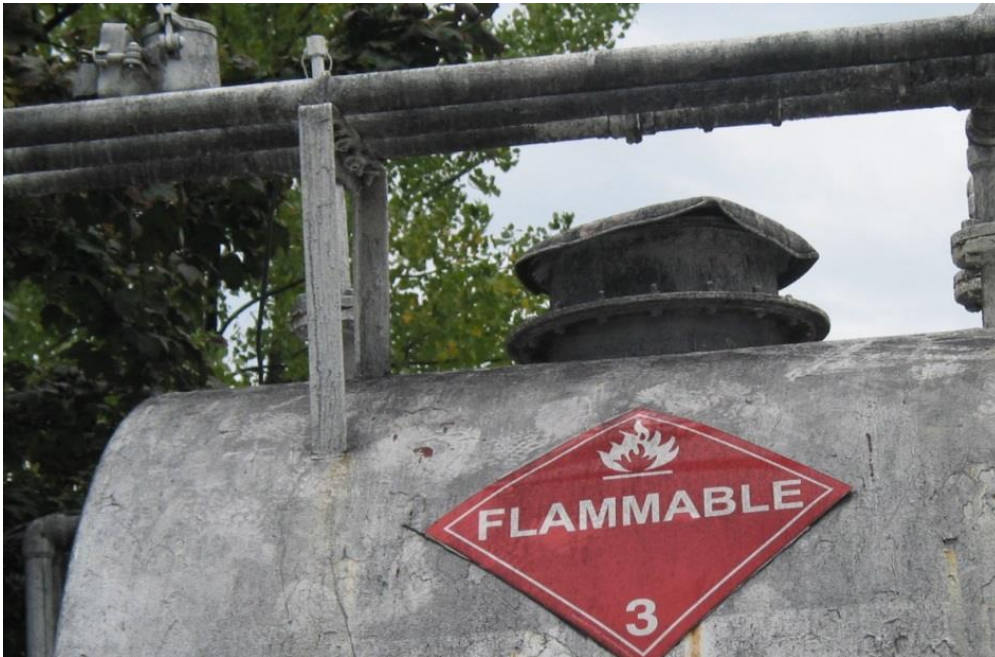
FIGURE 2. View of access port on top of tank.
