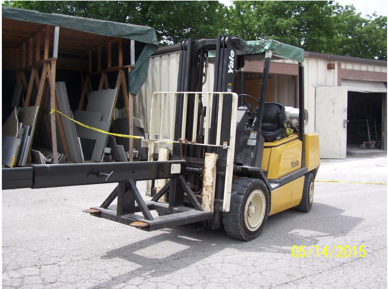
Photo #1: Forklift and boom used
