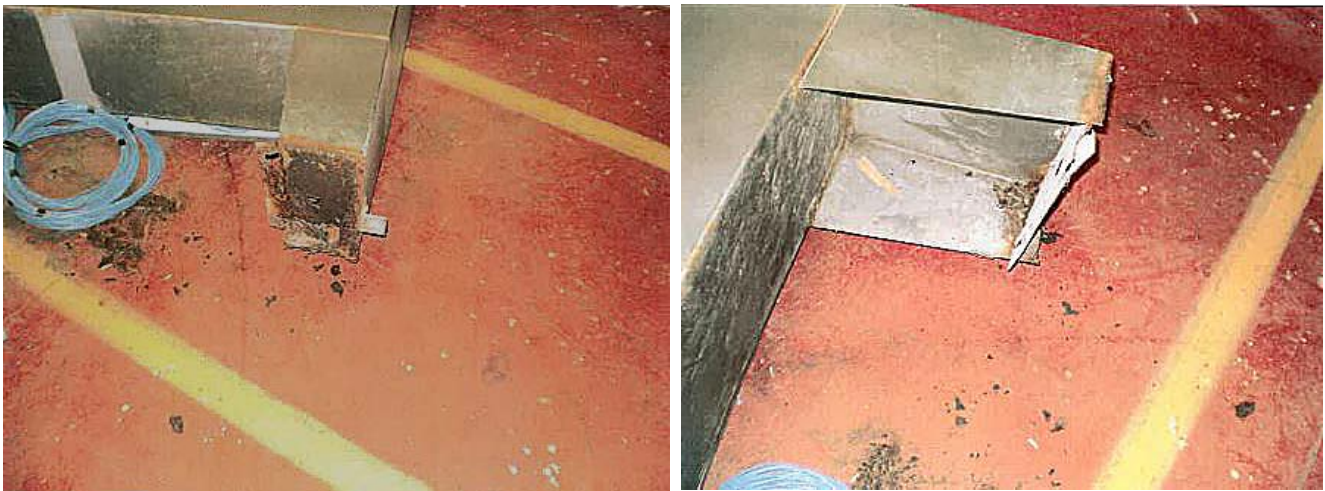
FIGURE 3. Views of cabinet foot at incident scene.
