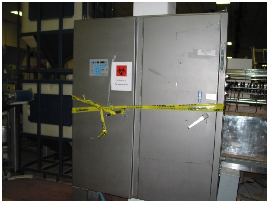
FIGURE 1: Front view of electrical cabinet upright.
