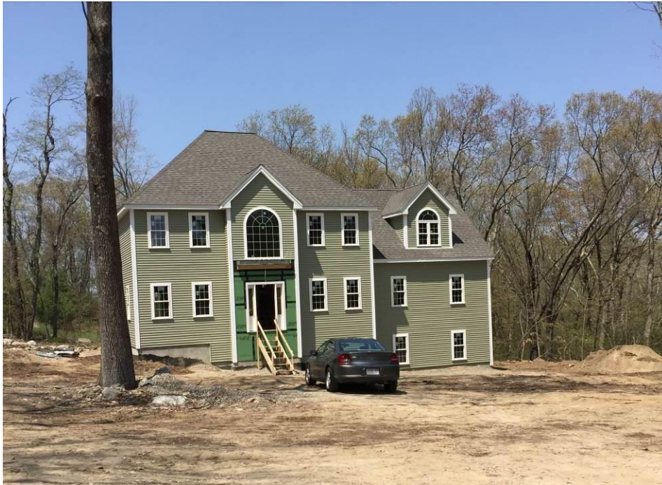
Figure 1 – The house being constructed at the time of the incident
