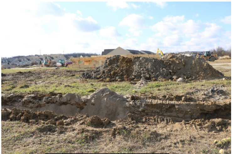
Figure 1. Placement of spoils
