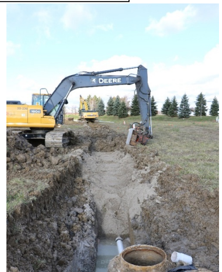
Figure 2. Water location in trench
