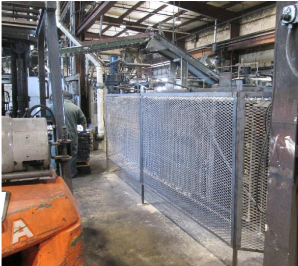
Photo 4. Installed guard at festoon line (Photo courtesy of OR-OSHA).
