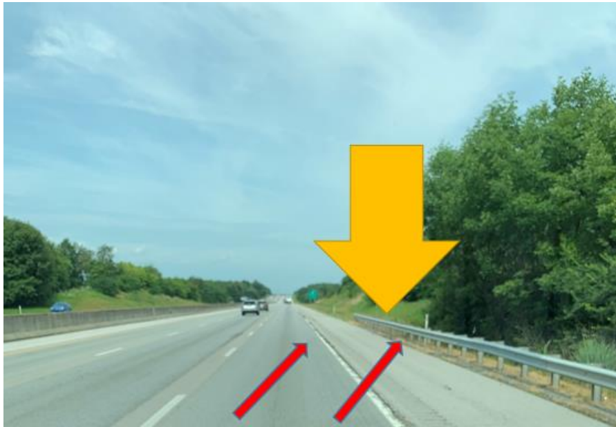
Photo 1. The RED arrows represent the initial path of the vehicle as it exited the travel portion of the roadway. The YELLOW arrow represents the first point of contact. (Vehicle vs. guardrail) Photo created by and property of KY FACE
