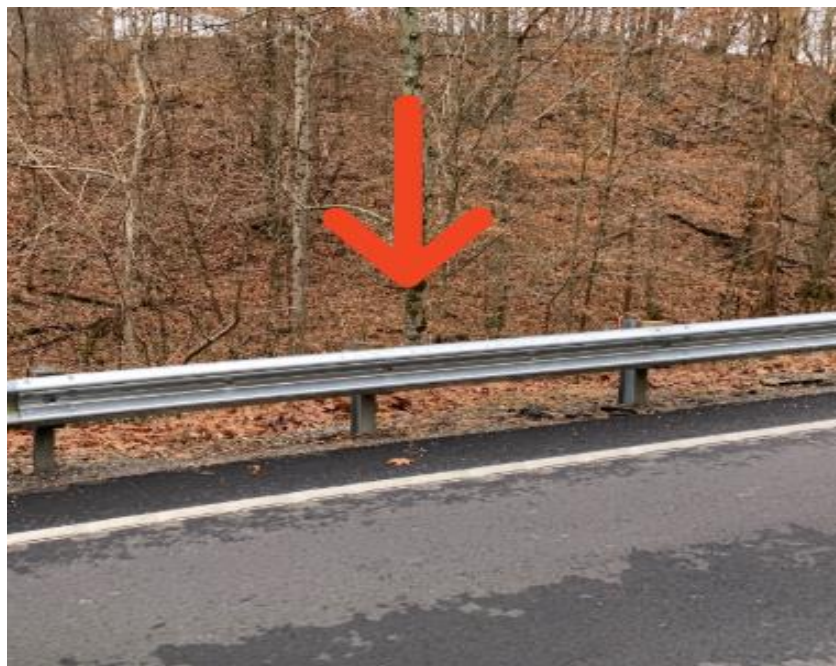
Photo 4. Photo of depicting the area the semi-truck and trailer overturned down the embankment. Photo by and property of KY FACE. (guardrail had been replaced when photos were taken)
