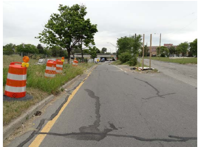
Photo 5. Construction materials at entrance ramp #2
