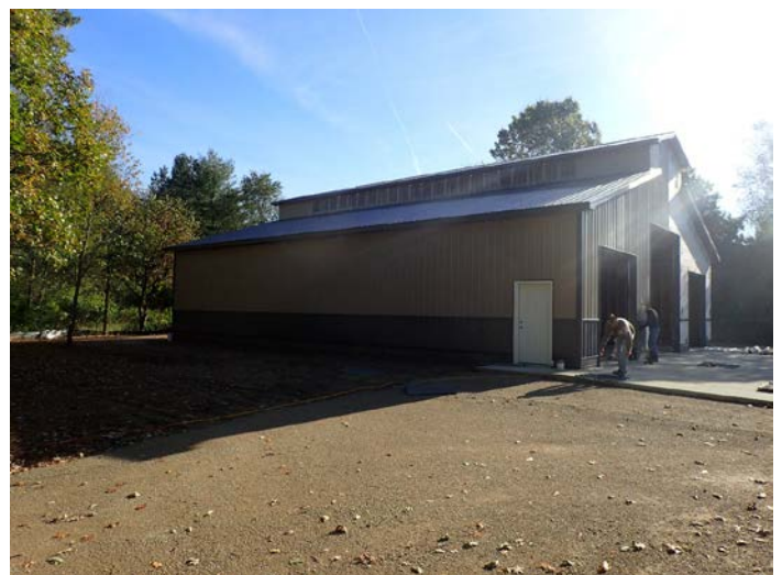
Photo 1. Pole barn under construction
