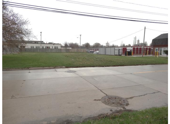
Photo 5. Driveway 1 no longer utilized as school entrance
