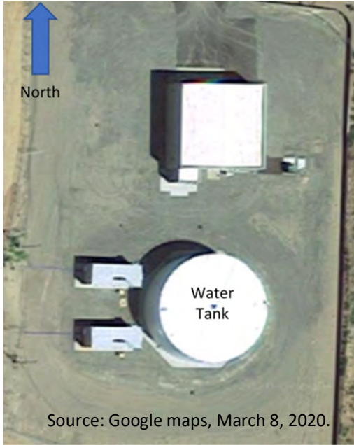
Photo 1. Incident scene, aerial view, after construction completed.
