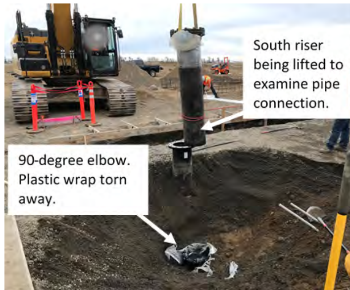
Photo 3. Post-incident excavation. South vertical riser to connection point with 90-degree elbow of horizontal pipe section. (Photo courtesy of OR-OSHA)
