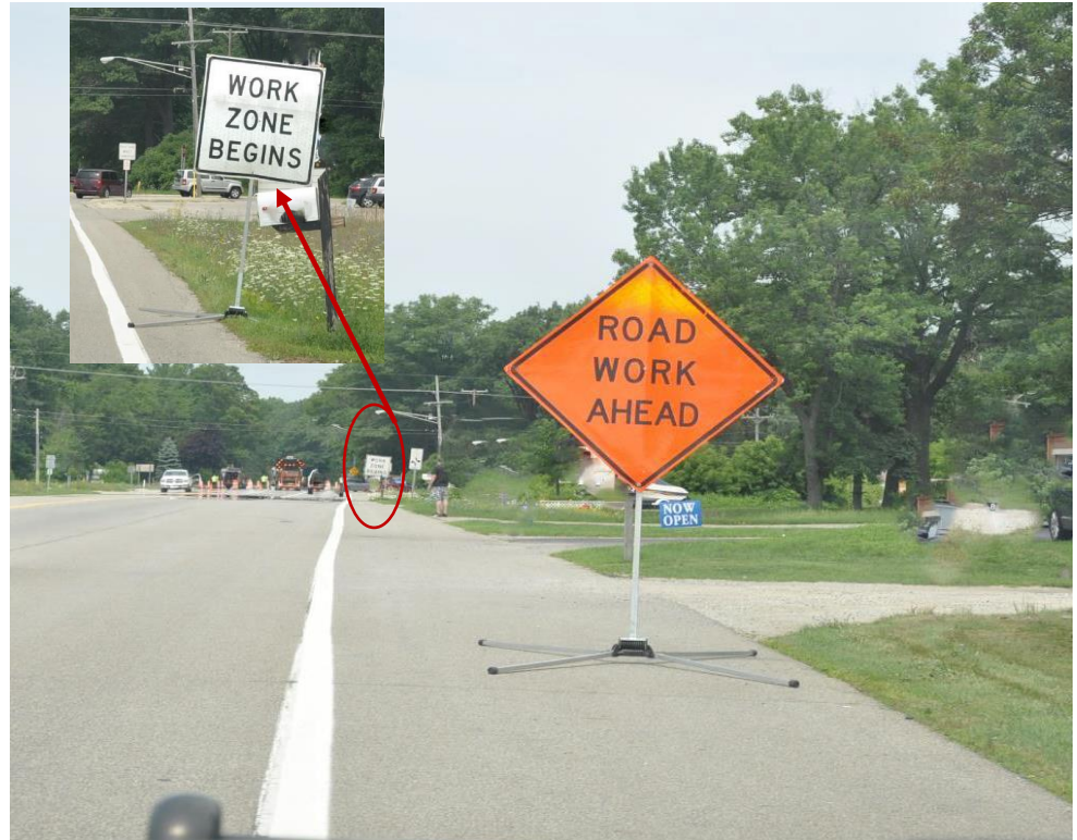
Photo 3. Road Work Ahead and Work Zone begins signs placed on northbound roadway, south of intersection
