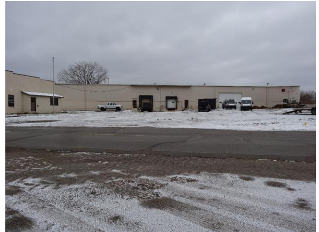
Photo 1. Warehouse undergoing demolition/renovation
