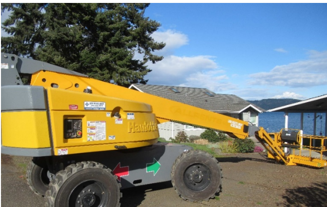
Photo 1: Incident scene driveway of residence with boom lift that workers were using to limb trees.
