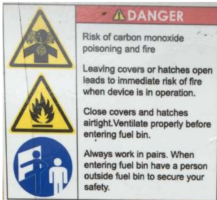
Figure 5 - Warning decal on the boiler/furnace and image of warnings listed on the decal on the boiler and on the hopper.
