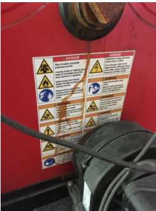
Figure 5 - Warning decal on the boiler/furnace and image of warnings listed on the decal on the boiler and on the hopper.
