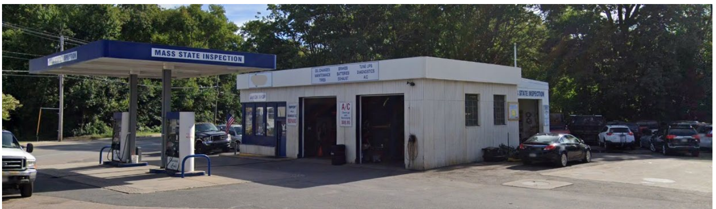
Figure 5 – Gas and service station; the incident occurred at the rear of the service bays (image from google maps)
