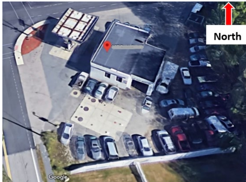
Figure 4 – Gas and service station; the inspection bay entry is visible on this side of the building (image from google maps)
