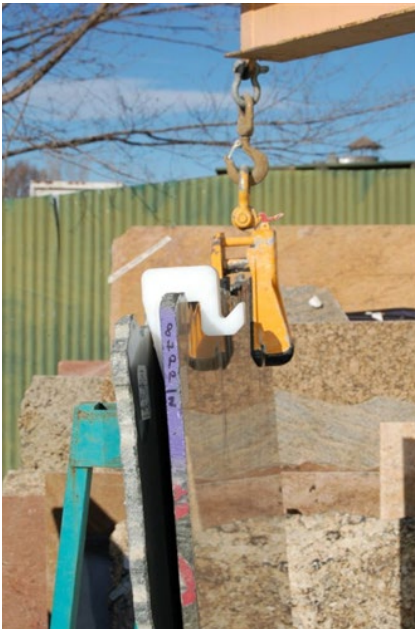
Photo 6: Positioning Relative to Rack [Wehause.com]
