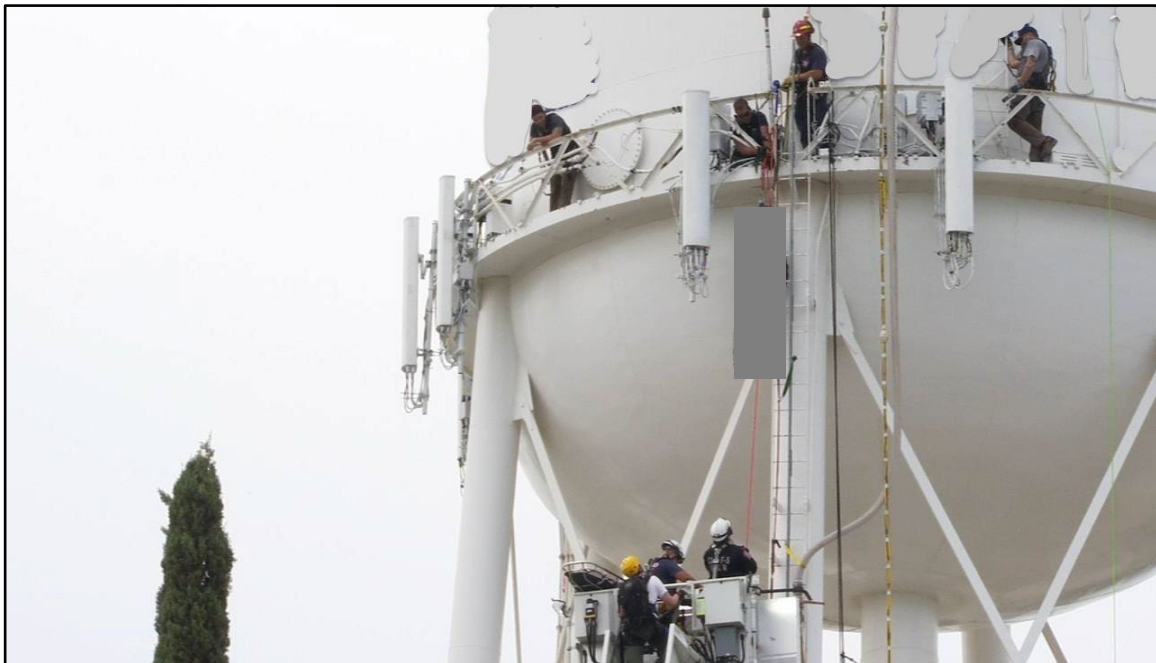
Exhibit # 2. Rescuers lowering the victim from the catwalk (photo courtesy ABC30).
