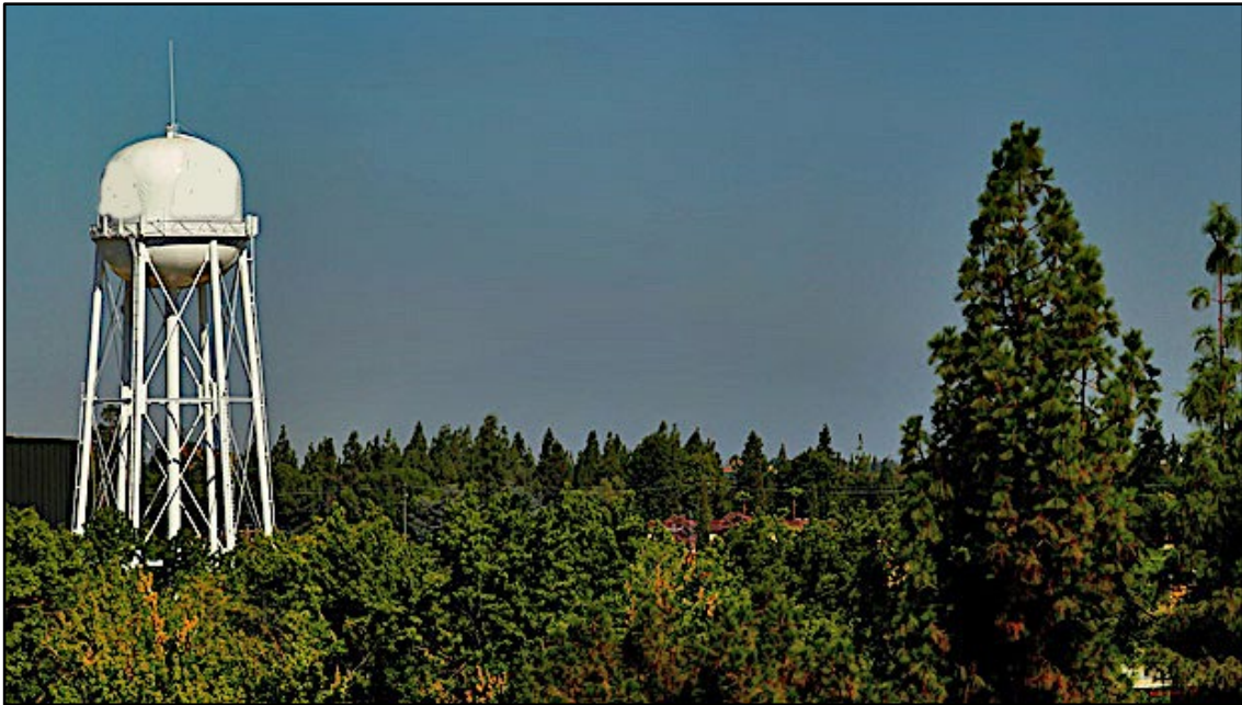
Exhibit 1. The 150-foot water tower being serviced.
