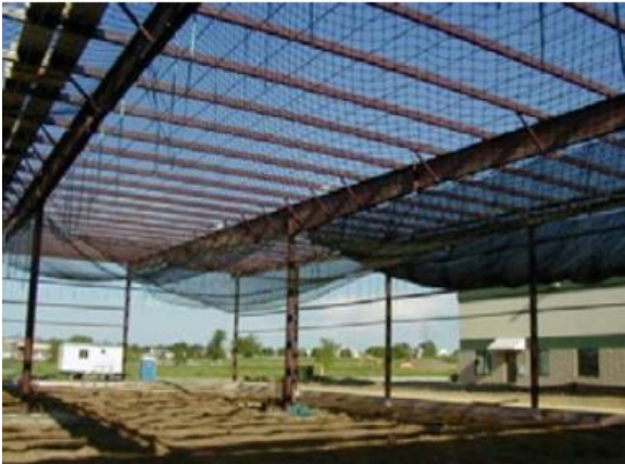
Photo 8. Safety net system [ OSHA, 2015 ]
