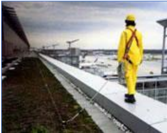
Photo 9. Personal fall arrest system [ OSHA, n.d. ]
