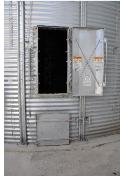
Exhibit 3 –Silo Access Door.
