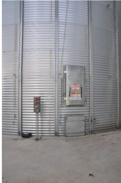
Exhibit 2 –Silo access door.
