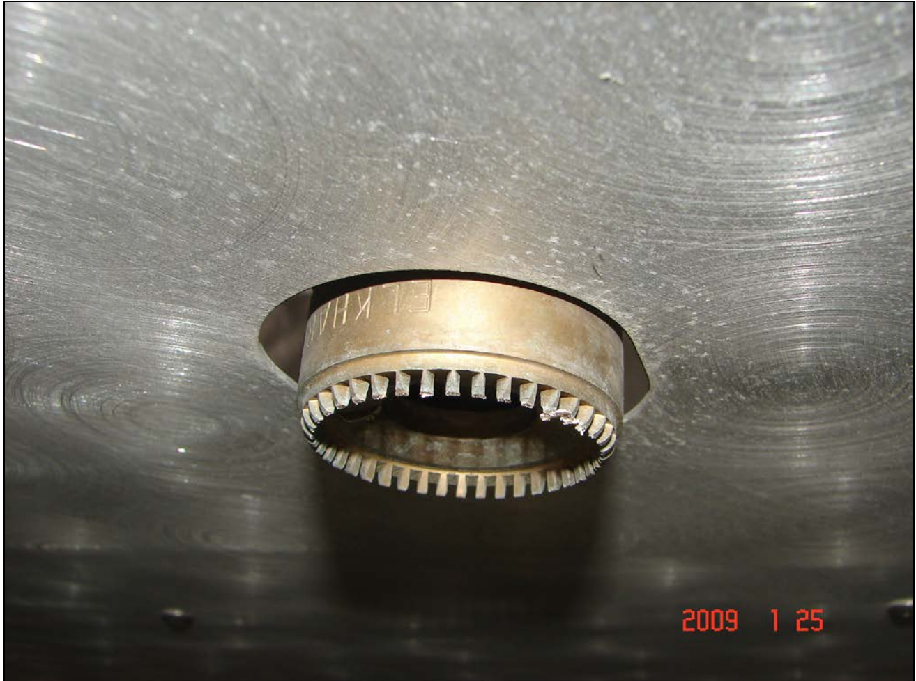
Photo 10. Bits of concrete debris on water curtain nozzle located at bottom of platform. Photo courtesy of police department.
