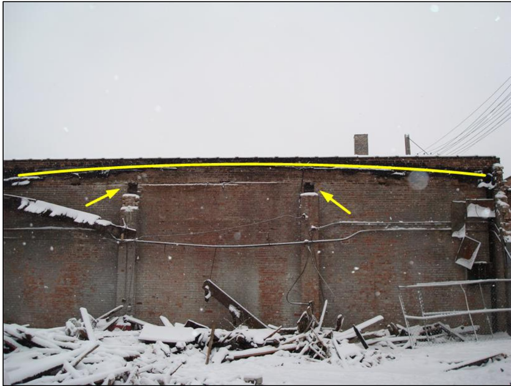
Photo 2. Photo shows the Sector 2 wall that supported western end of the bowstring truss roof. The two arrows indicate the truss-end pockets in the brick masonry wall at the top of the brick pilasters where the ends of the two bowstring trusses rested. The roof was supported in the middle by the two bowstring trusses while the north and south ends were supported by the front and rear non-load bearing walls. The line indicates the approximate curvature of the roof. (NIOSH photo)
