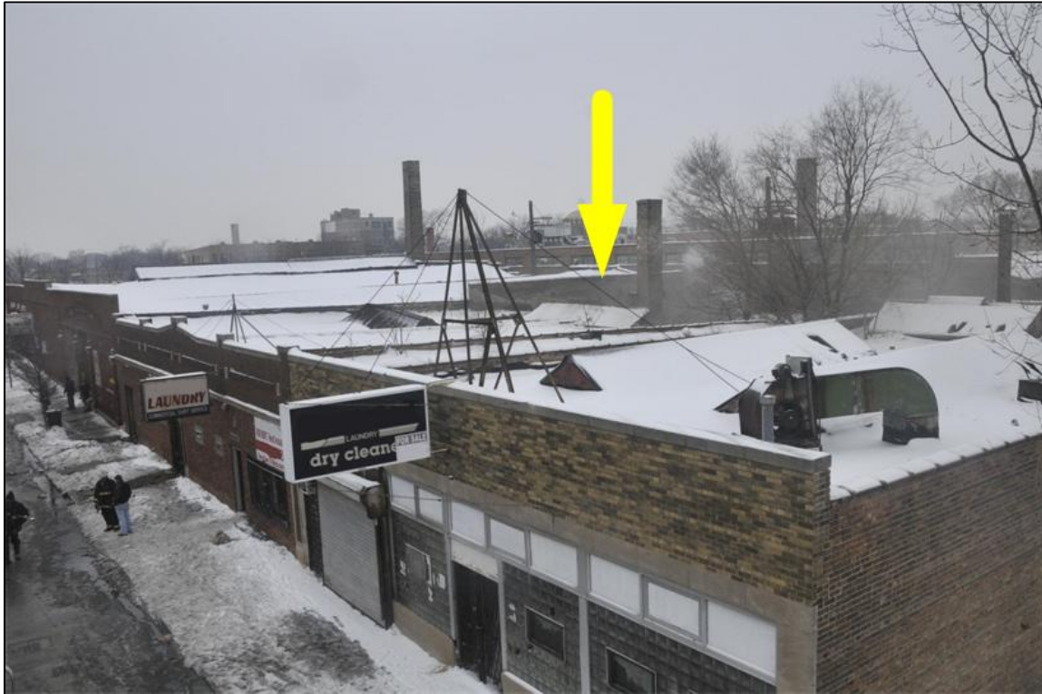
Photo 4. Elevated view of the block where the incident occurred, taken the day of the fire. The arrow marks the location of the collapse. The photo has been edited to remove names and identifying information from signs. (Photo courtesy of fire department)
