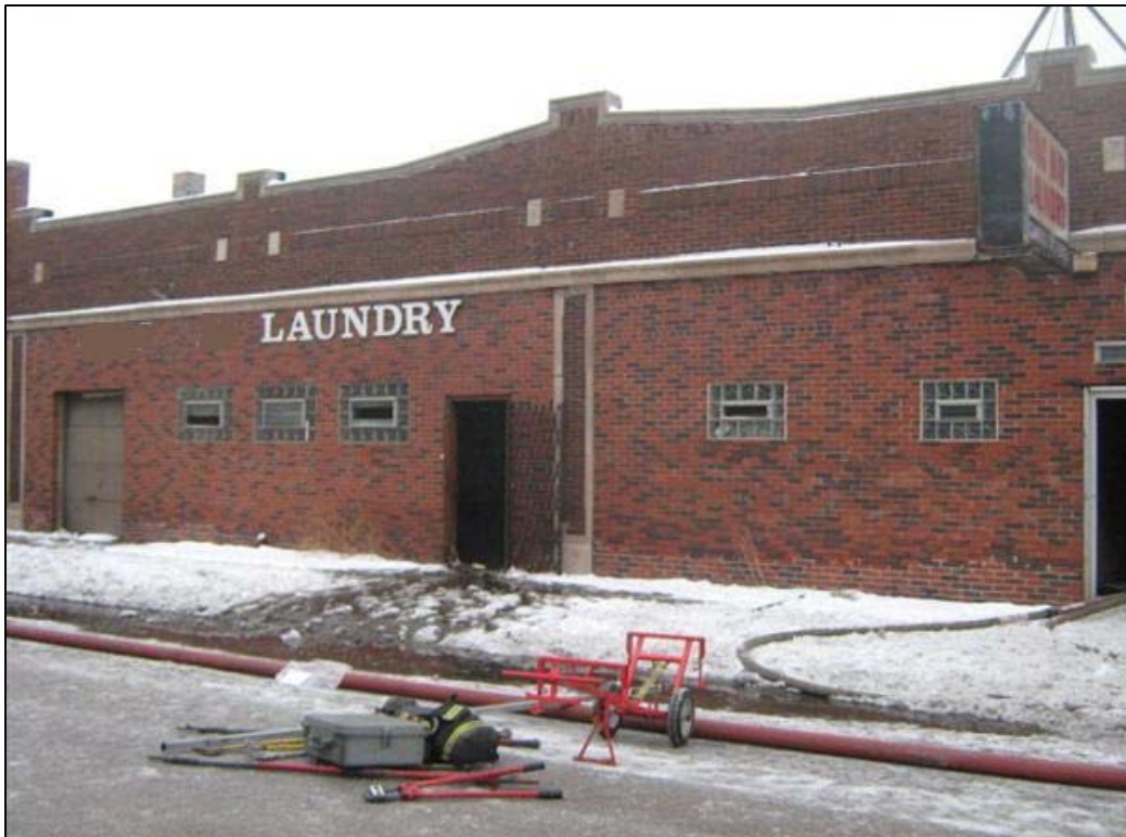
Photo 5. Front view of structure as viewed from the street (Sector 1). Buildings along the street appeared to be in good condition from this view. The deteriorated condition of the roof was not visible from street level. Photo taken the day of the incident. (Photo courtesy of city Department of Buildings)
