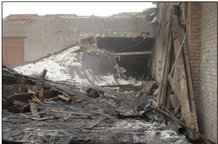
Collapse scene as viewed from building rear facing building front. Note portion of bowstring truss leaning against wall at right side of photo. (Photo courtesy of fire department)
