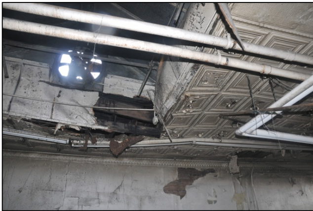
Photo 6 and Photo 7. Photo 6 (left) and Photo 7 (right) show the deteriorated ceiling conditions inside the front part of the structure. (Photos courtesy of fire department)
