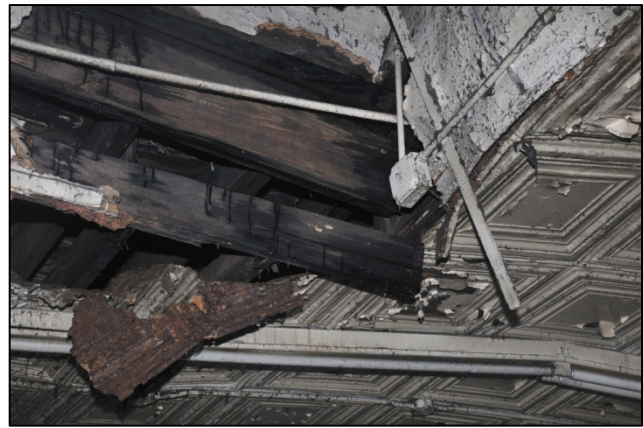
Photo 6 and Photo 7. Photo 6 (left) and Photo 7 (right) show the deteriorated ceiling conditions inside the front part of the structure. (Photos courtesy of fire department)
