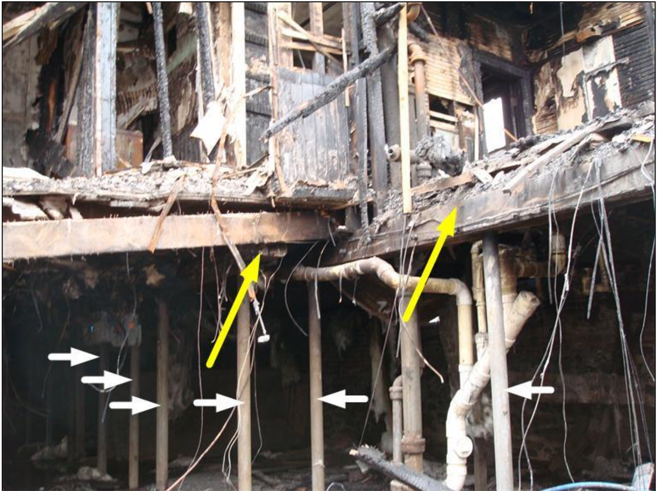
Photo 4. Yellow arrows indicate the two heavy timber support beams running front to rear and located near the center of the structure. White arrows indicate tubular metal support posts commonly referred to as lally columns or lally posts. Note the off-set between the two support posts as indicated by the two supports at the lower center of the photograph.
