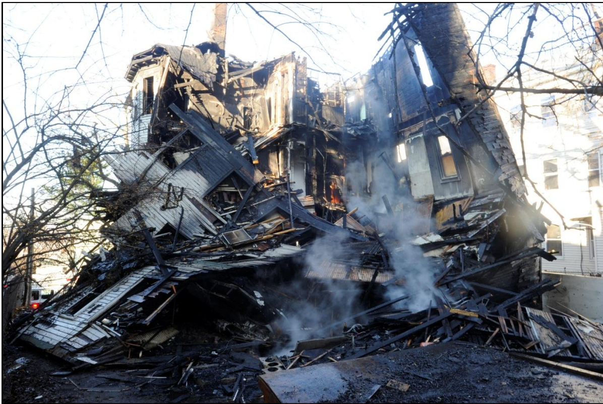
Photo 5. Photo taken from the rear of the structure just hours after the collapse. The left side of photo shows the remains of the collapsed portion of the Side D wall. (Photo courtesy of the State Fire Marshal's Office)
