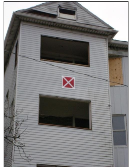
Hazardous building placard attached to exposure structure located just south of the fire building. (NIOSH Photo)
