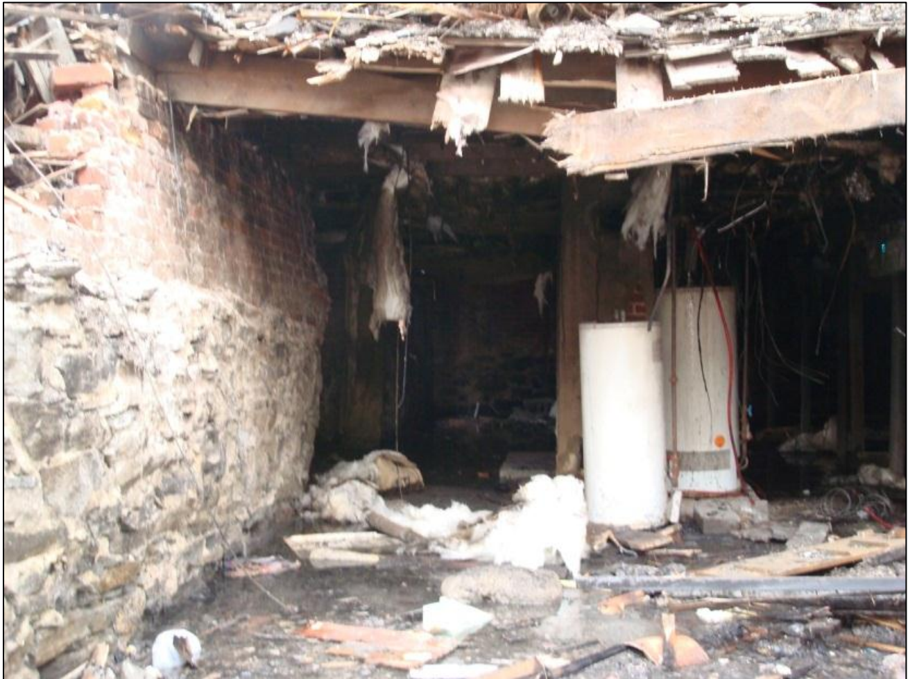
Photo 2. View of the D-side basement wall. Note the brick and mortar wall laid over top of the field stone. View is close to the area where the injured fire fighter was extricated. (NIOSH Photo)
