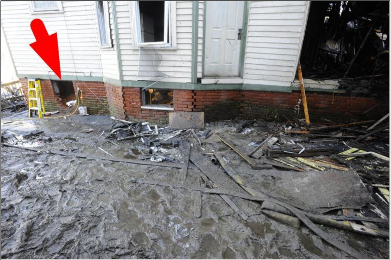
Photo 7. Arrow marks location where foundation wall was breeched to access the cellar to extricate the injured fire fighter.
