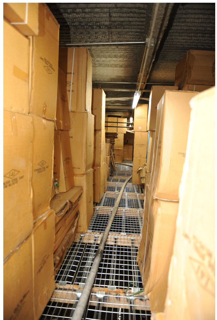
Photo 3. Hoseline stretched down the “catwalk”. The attack line was stretched down the catwalk leading to the fire area.
