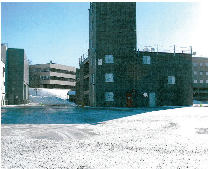
Photo 1: Fire Department Training Center's Tower B Photo by Anchorage Fire Department.
