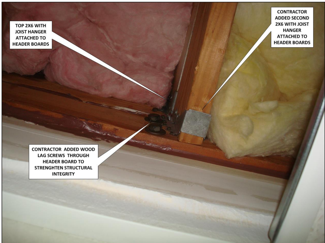
Photo 4. Double 2x6 floor joists and lag screws added by contractor in an attempt to improve structural integrity within the apartment complex.
