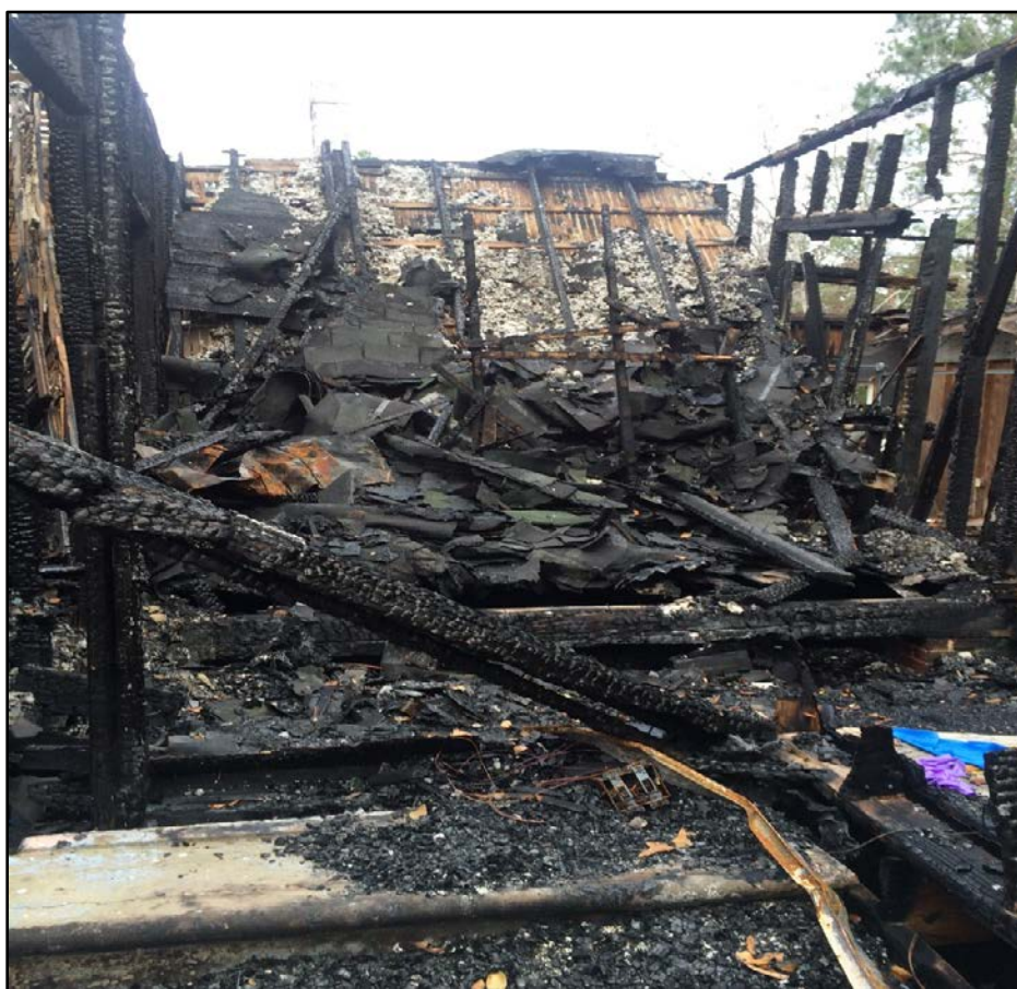
Photo 6. Example photo of ceiling load in adjacent room. (NIOSH photo.)
