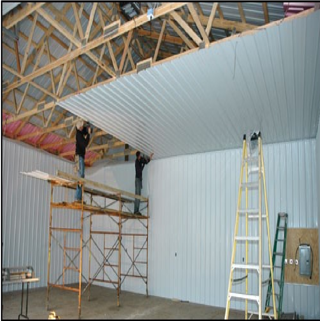
Photo 1. Similar roof and pan ceiling construction. (Photo courtesy of Chief Brian Kazmierzak)
