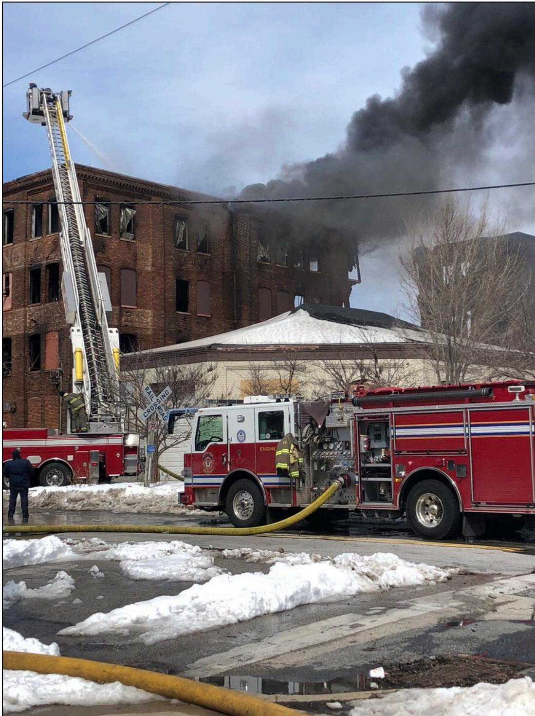
Photo 6. Photo shows defensive master stream operation on March 22, 2018 at Side Alpha / Delta corner.
