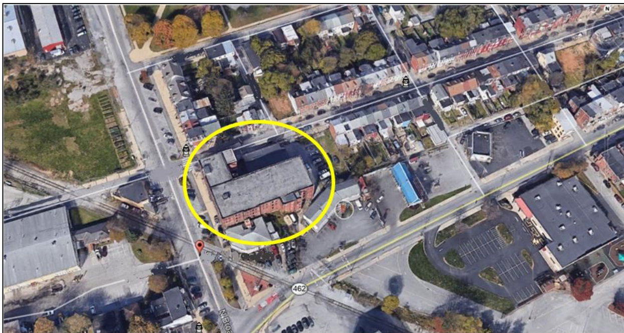
Photo 1. Overhead view of four-story Type IV (heavy timber) commercial mill structure where the incident occurred. Structure is highlighted in yellow. (Photo adapted from Google Earth satellite view)
