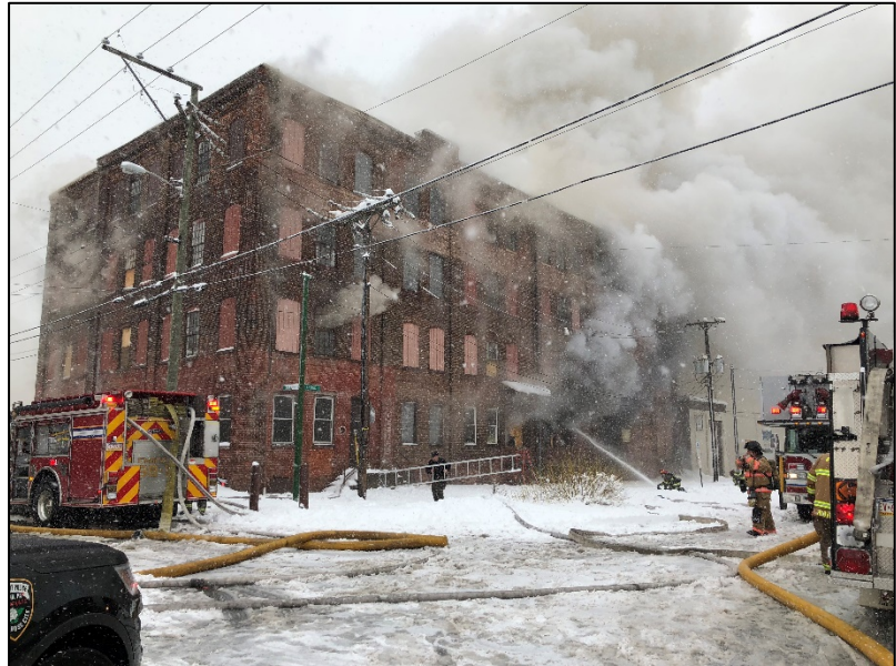
Crews work on Side Alpha on March 21, 2018 at 140-year old mill building. Time is approximately 1642 hours. Two fire fighters died following collapse on March 22, 2018.
