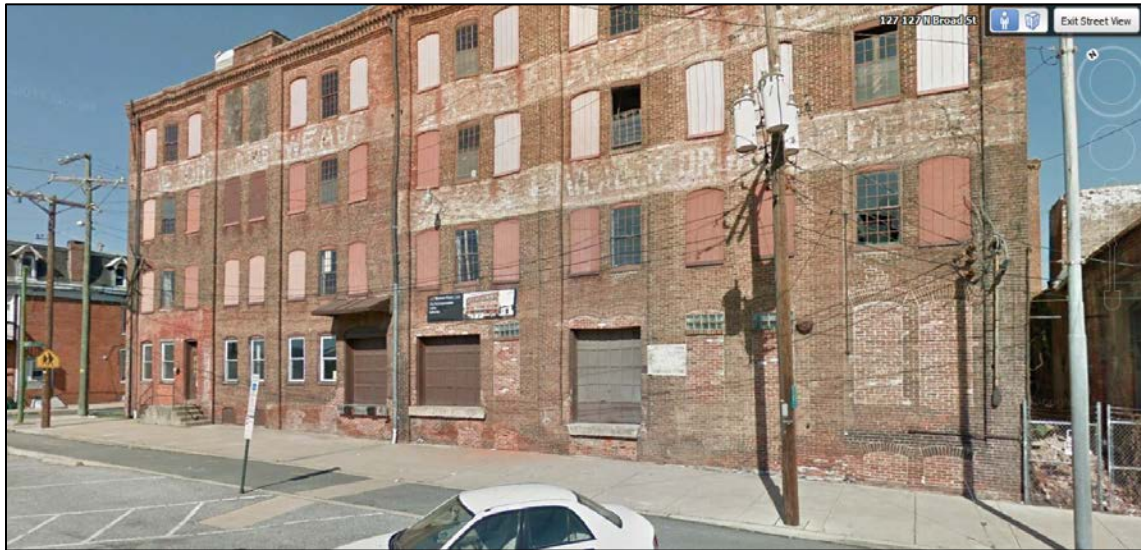
Photo 2. Side Alpha view of structure before the fire. Initial attack crews entered the structure through the man door at the Side Alpha / Bravo corner. (Photo adapted from Google Earth street view.)
