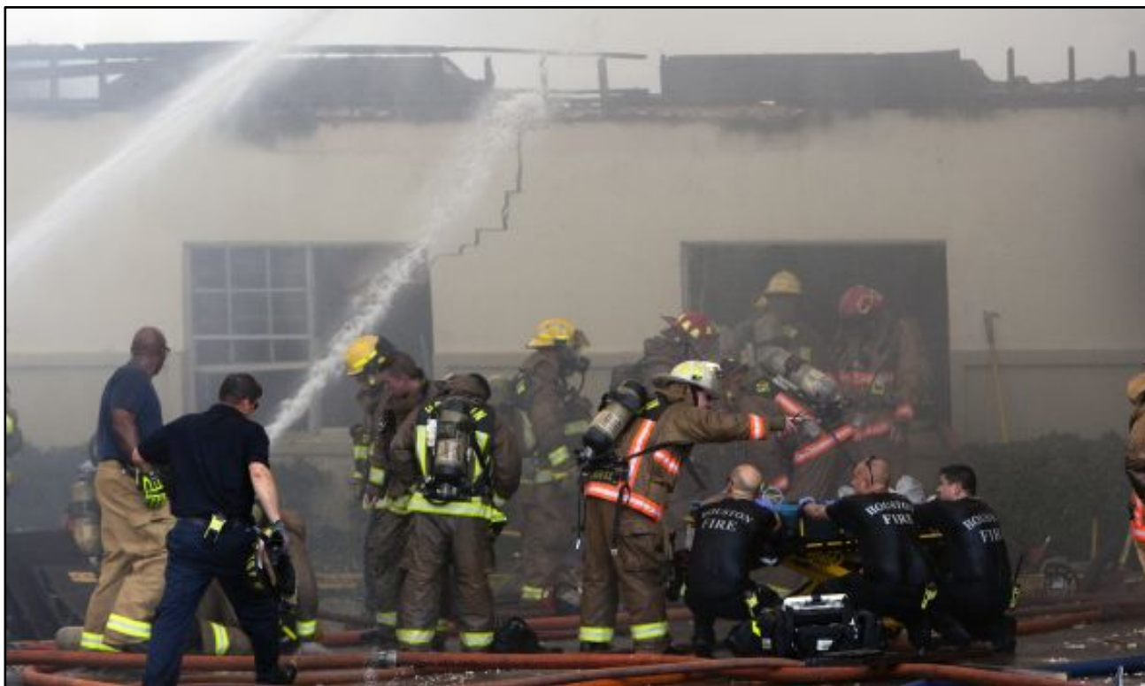
Photo 6. A 20 ft. x 8 ft. foot section (160 SF) of compromised perimeter wall collapse into the immediate area directly in front of the structure. Three members from the Rescue Group became trapped under falling debris that resulted from the secondary collapse. These firefighters were quickly removed by other members in the immediate area and then taken to awaiting EMS crews. The time is approximately 1225 hours.
