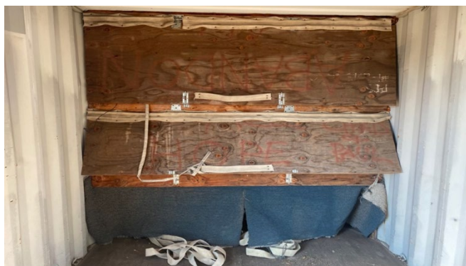
Figure 3. Maze with closed emergency access doors to middle and top levels and skirting lowered at bottom level. Photo by NIOSH.
