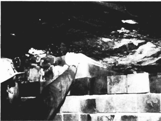
Figure 12.—Wedging of wood blocks to mine roof.
