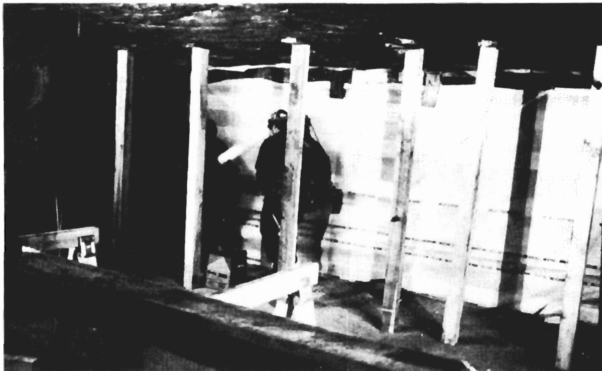
Figure 8.—Wooden framework for cementitious foam seal.
