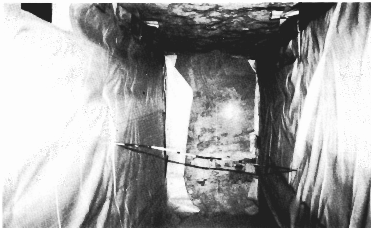
Figure 9.—Brattice liner attached to framework used to contain the cementitious foam slurry. Note copper tubing through the middle of the seal.
