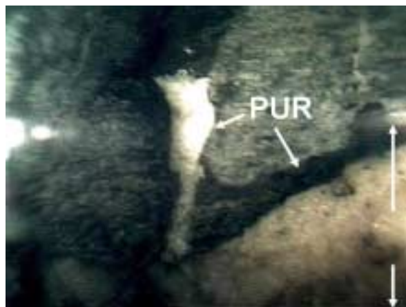
Figure 7. PUR filling fractures at 1 ft into the roof at intersection No. 32.
