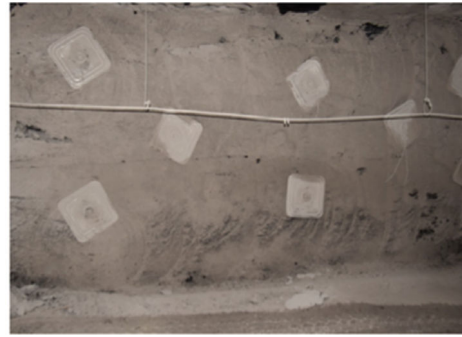
Fig. 2. Typical rib support pattern at site-1 for a mining height of more than 2.1 m.
