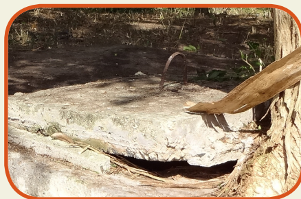
Repair broken septic tank covers
