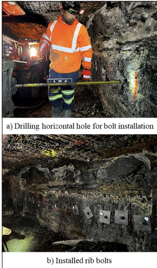
Figure 3. SEPTs preparation carried out at the NIOSH Safety Research Mine
