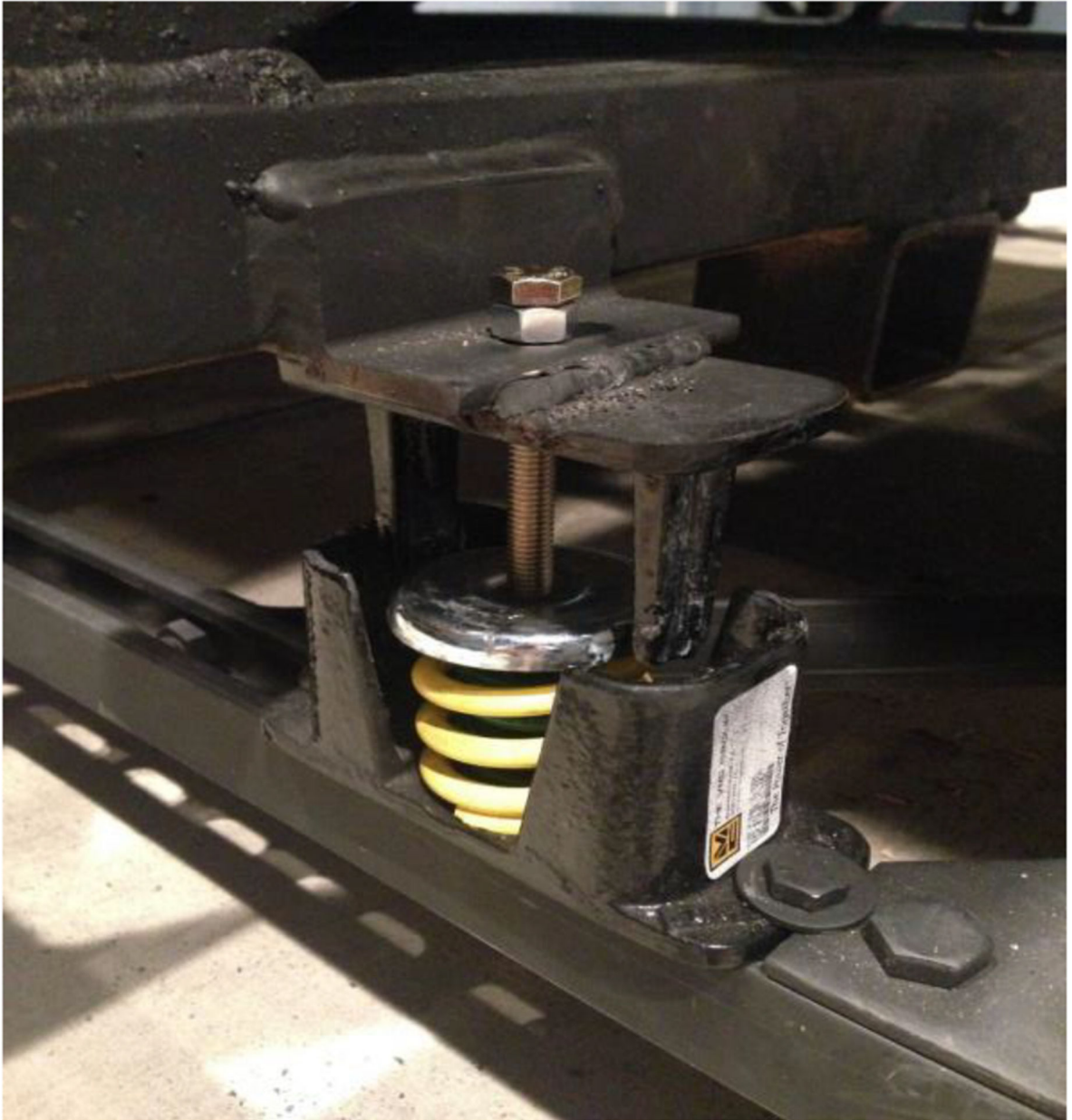
Figure 3. One of the four extreme mount spring-dampers exhibiting a stiffness of 520 pounds (236 kilograms) per 0.75 inches (1.9 centimeters) of compression
