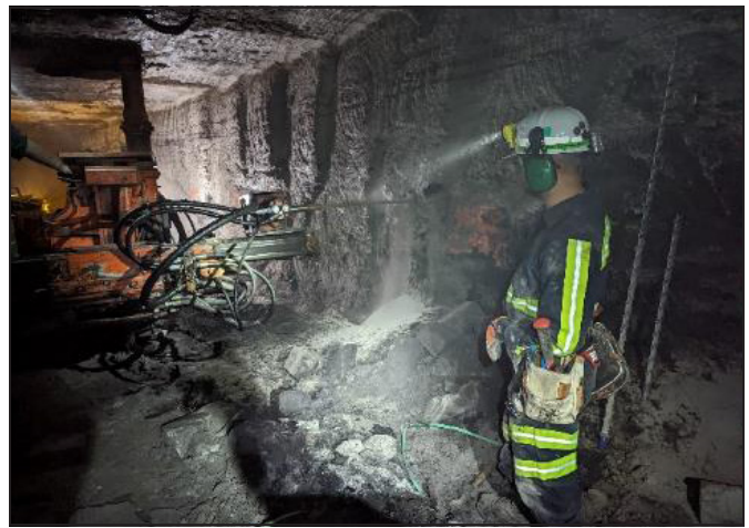
Figure 4. Example of drilling operations resulting in the production of dust
