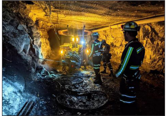
Figure 16. Example of some slip, trip, and fall hazards including wet and uneven terrain, water line, rib sloughage
