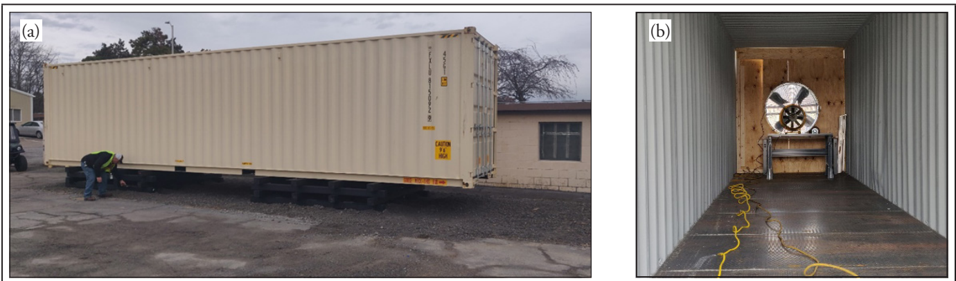
Figure 1. Steel shipping container (a) outside and (b) inside, modified to be used as a fire suppression test facility
