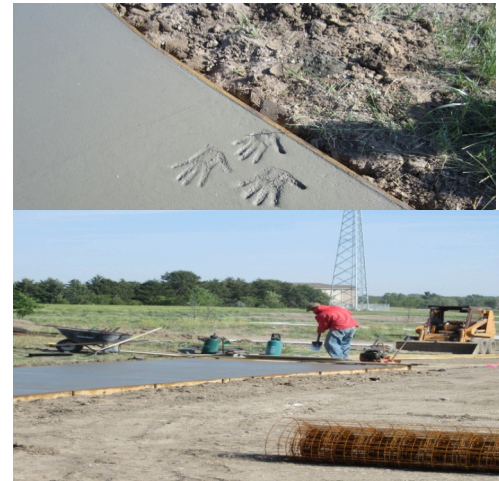
Phase one construction of two-mile community walking trail in Colby, KS
