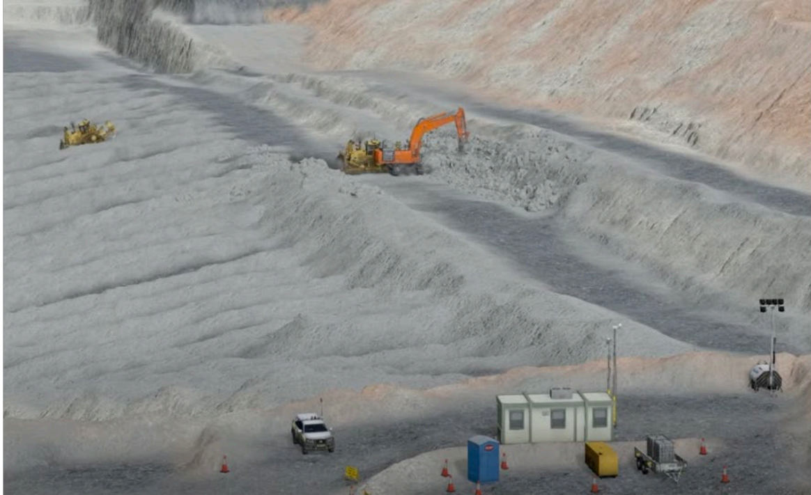
Figure 7: Overview of the collision between a semi-autonomous dozer (DZ2003) and excavator that occurred at Wilpinjong mine in 2019. ( https://www.youtube.com/watch?v=zLqxdVa66qY ).
