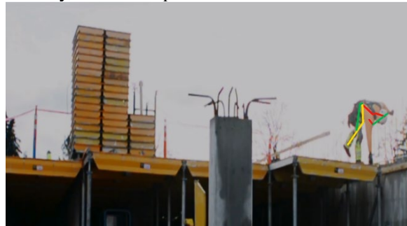
h. Hammer a modular panel in place
