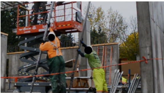
m. Hold a shoring post in place
