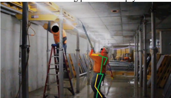
e. Loosen a modular panel with a pry bar
