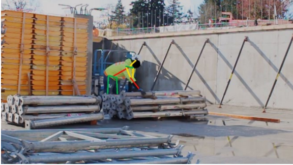
i. Adjust the height of a shoring post by hand
