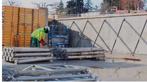
j. Inspect with a tape measure
