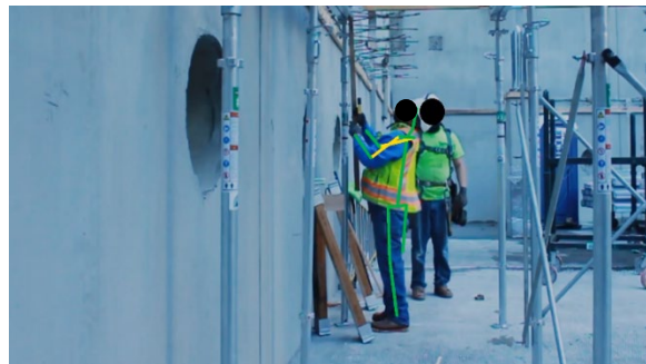
n. Inspect with a level
