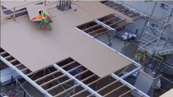
c. Carry a sheathing panel
