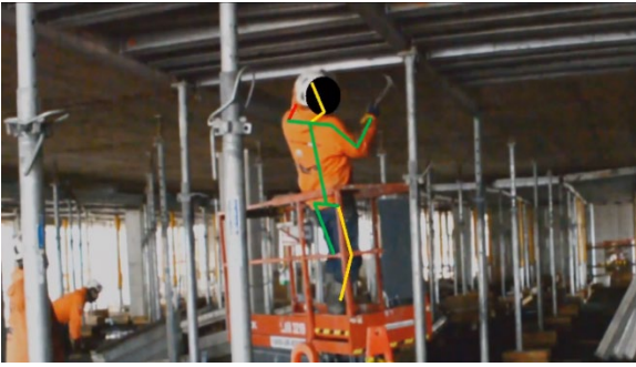
a. Loosen formwork connection with a hammer
