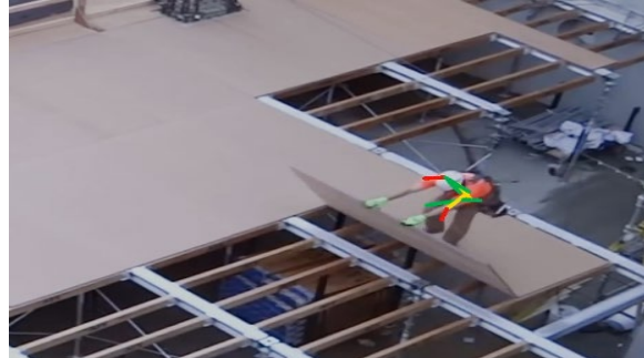
d. Place a sheathing panel
