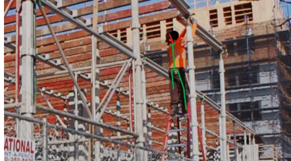
b. Lift a main beam
