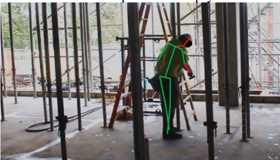
g. Loosen a shoring post connection with a hammer
