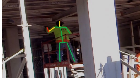
b. Lower a secondary beam
