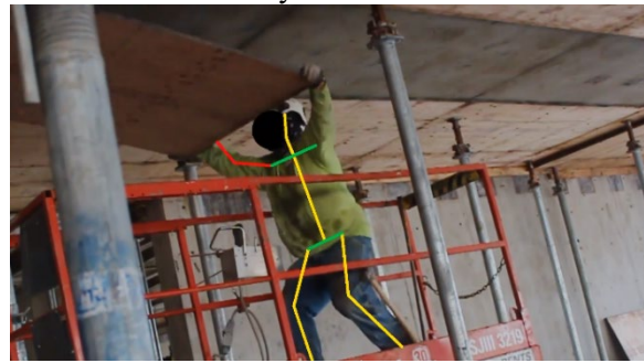
d. Loosen a sheathing panel by hand
