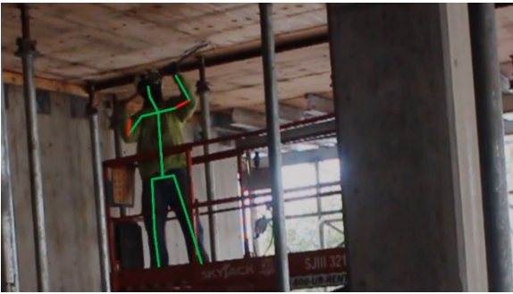
c. Loosen a sheathing panel with a pry bar
