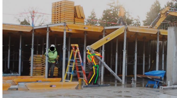
l. Plumb a shoring post
