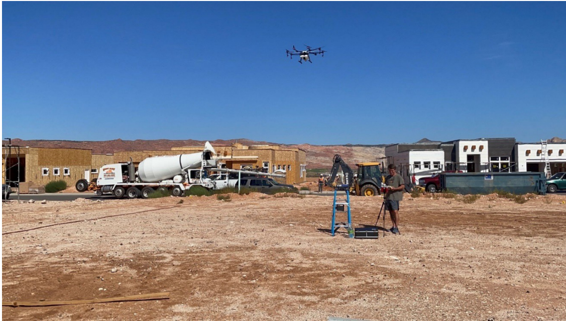
Figure 6 – Multiple construction activities going on during site sampling events.
