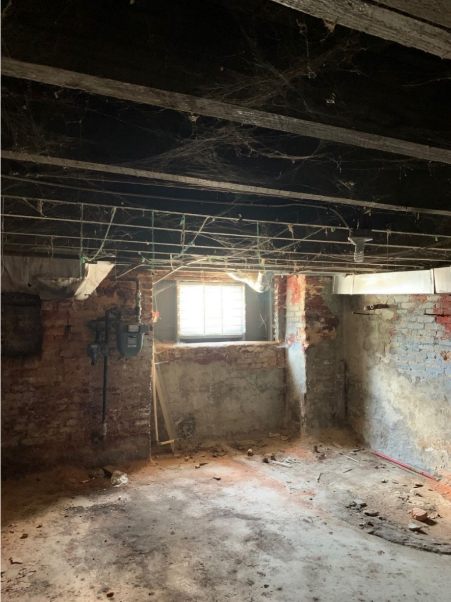
Photo 4: Basement Walls, HVAC, and a Window
