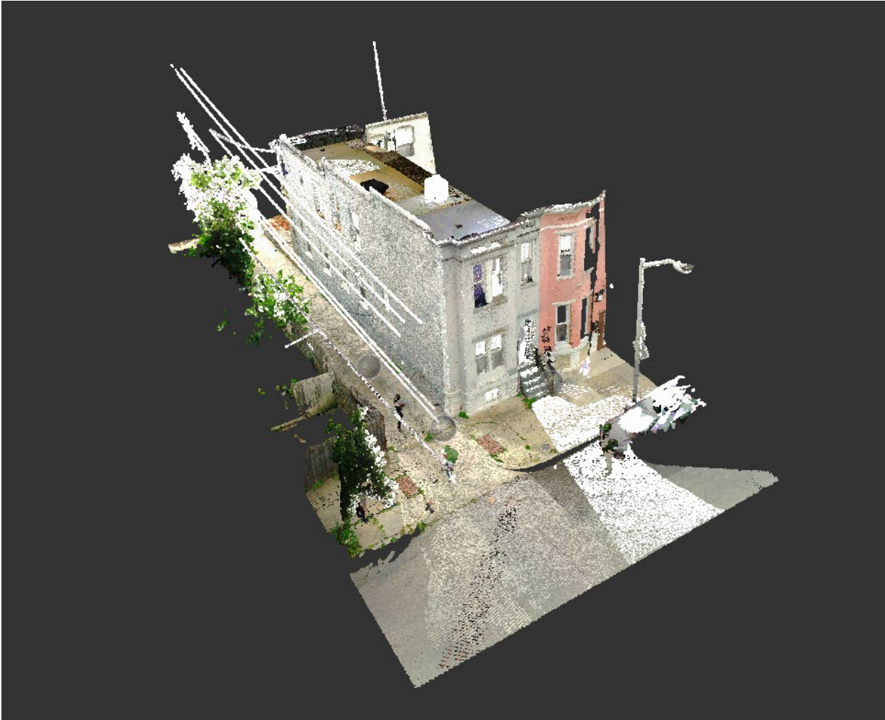
Model 1: Point Cloud Data of the Building from the Front
