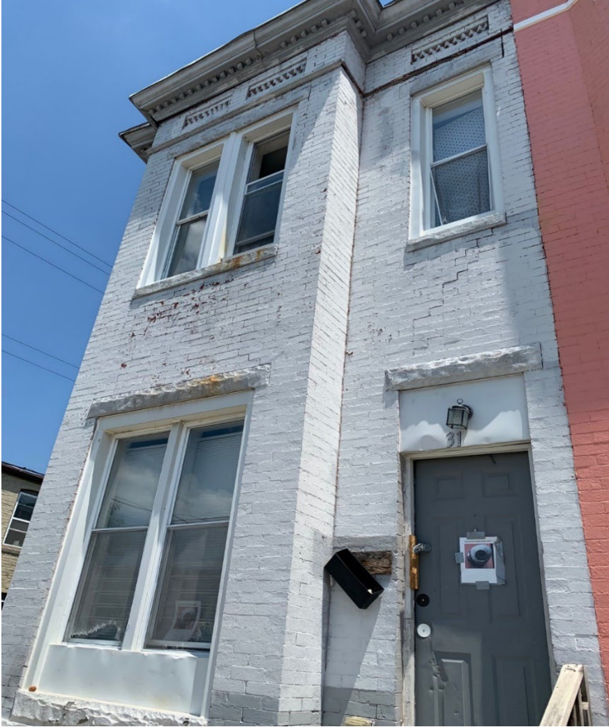
Photo 1: Front Brick Façade of the Row House
