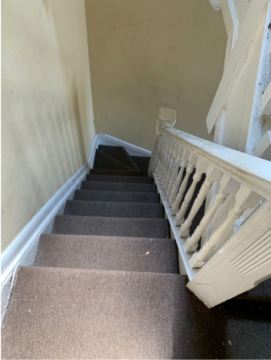
Photo 6: Narrow Stair Leading to the Second Floor from the First Floor
