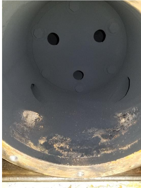
Figure 48 - Exhaust Baffle Plate Post-Test
