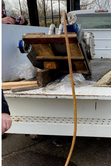
Figure 131 - Exhaust Side Hydrostatic Test
