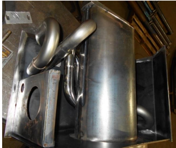
Figure 32 - Exhaust Piping Fabrication
