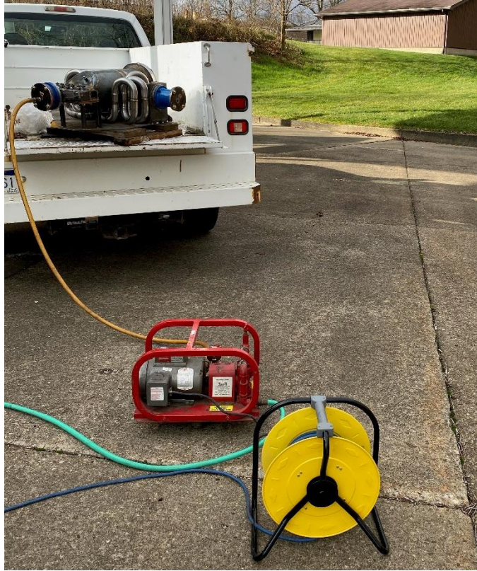
Figure 128 - Hydrostatic Test Apparatus During Intake Side Test
