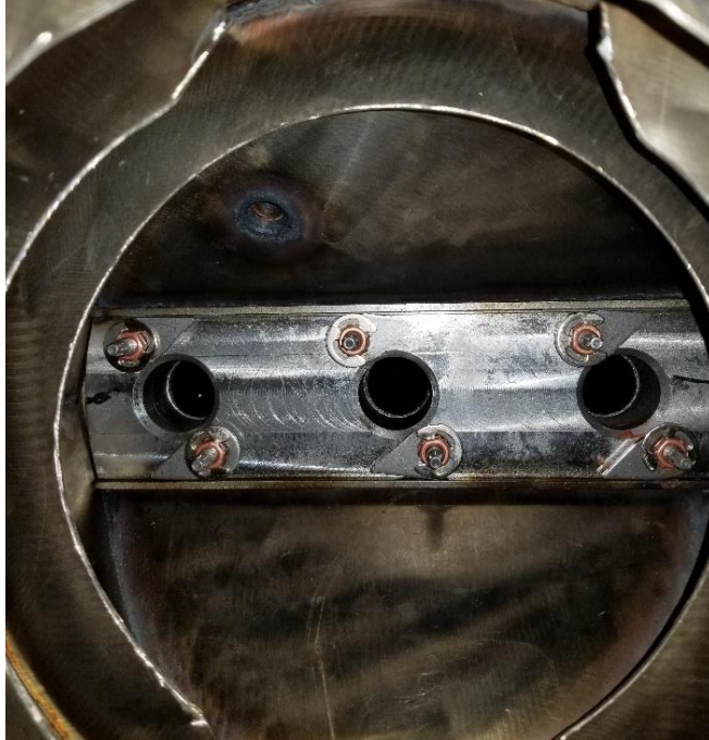
Figure 122 - Exhaust Manifold Installed
