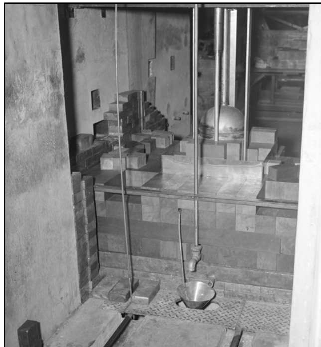
The “Water Boiler” reactor (shown here partially disassembled) used enriched uranium fuel in liquid form and was surrounded in part by beryllium oxide blocks.
