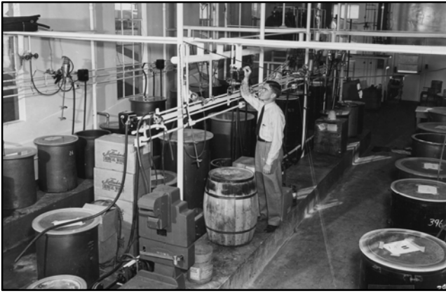
In this DP West Site solutions preparation room, chemicals were mixed in large vats and fed by gravity to operations below.
