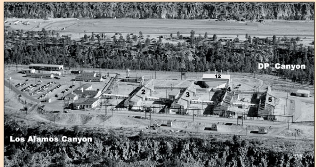
Fig. 2. DP West Site at what became known as TA-21 took over plutonium production late in 1945. Process exhaust from Buildings 2, 3, 4, and 5 was collected, treated, sampled, and released via four main stacks at Building 12.
