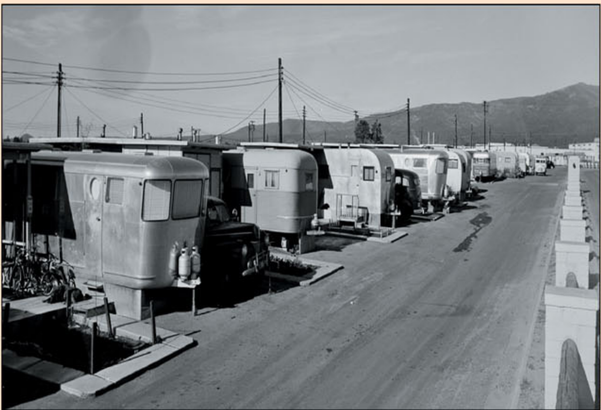
Fig. 10. The trailer park located 1 km west of the DP West Building 12.
