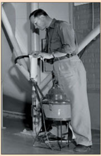
Fig. 4. A modified "Filter Queen" vacuum cleaner used for stack sampling at DP West Site at Los Alamos.
