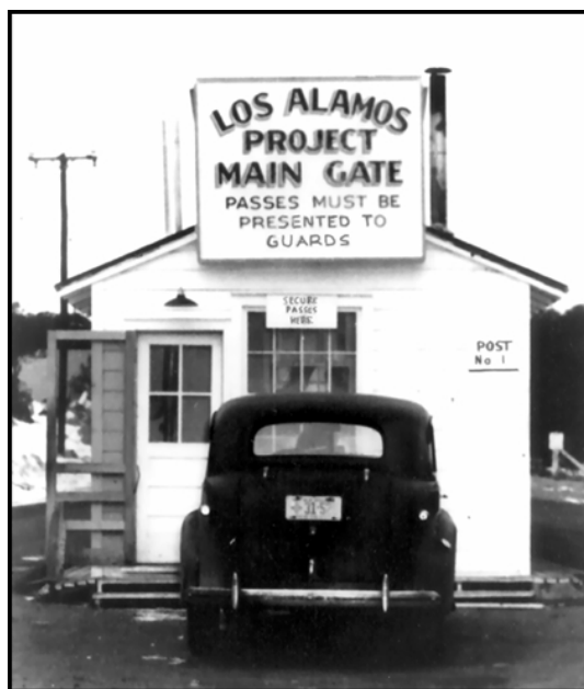
Figure1-4: An early photo of the main gate into LANL
