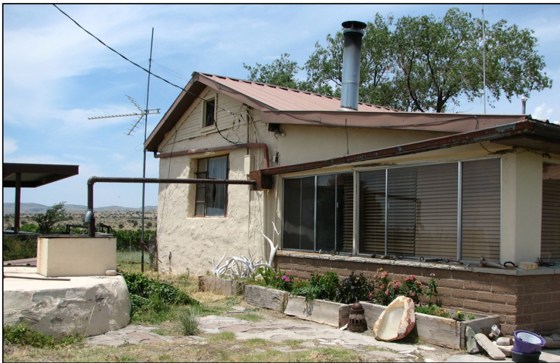
Fig. 10-20. A system for collection of water off the roof of a residence on the Black Hills Ranch, formerly the Nalda Ranch, east-northeast of the Trinity Site. The cistern to the left, which was damaged by the Trinity blast and then repaired, is still in use today.
