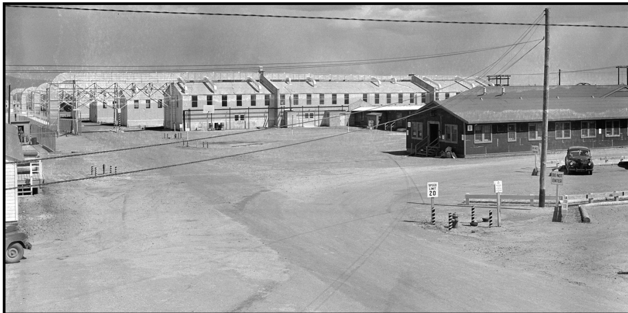
Fig. 4-19. Primary buildings of DP West on 16 May 1947. Photo courtesy of LANL (IM-9: 05426)
